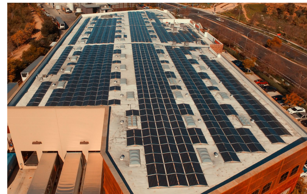
► D-Dome installation on Stone Brewing Co. in Escondido, CA.
